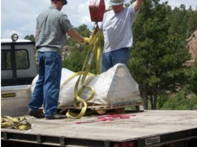
Unloading the incredibly well-built generator section
