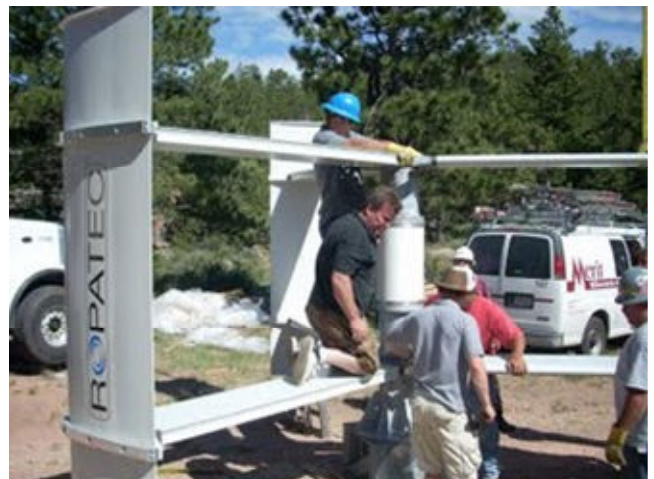
Final assembly on the ground
